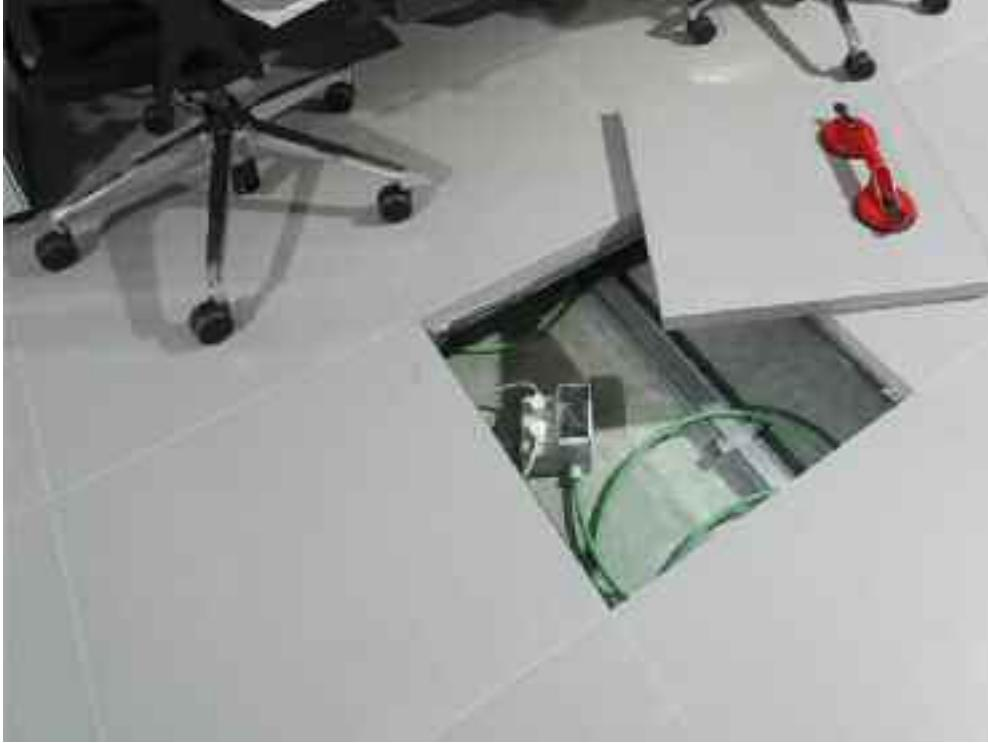
**Easiness** - Raised floors are carried out via dry installation, a quick and easy installation system.
