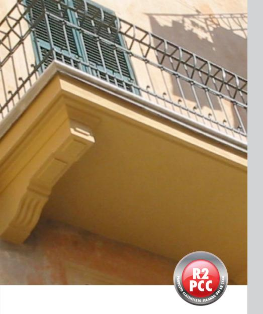
MALTA PREMISCELATA RAPIDA, DI TIPO PCC E CLASSE R2 SECONDO UNI EN 1504-3, ALTA-MENTE TISSOTROPICA, RESINATA E FIBRO-RINFORZATA, PER LA RICOSTRUZIONE VOLU-METRICA DEL CALCESTRUZZO.
