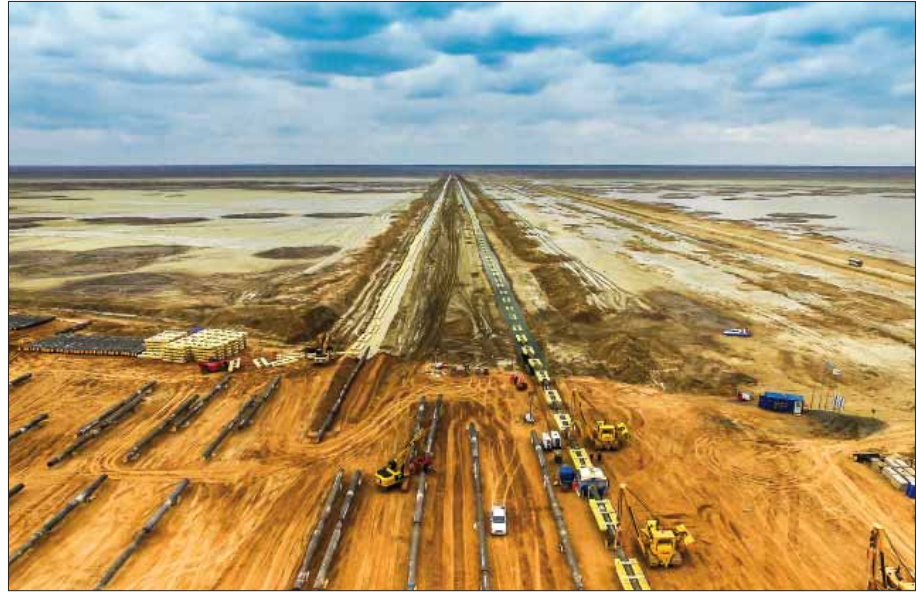
KAZAKISTAN BONATTI Kashagan Pipeline Replacement Project
