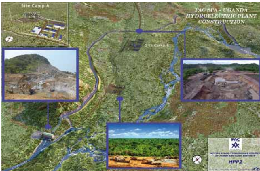
UGANDA PAC Hydroelectric Plant Construction
