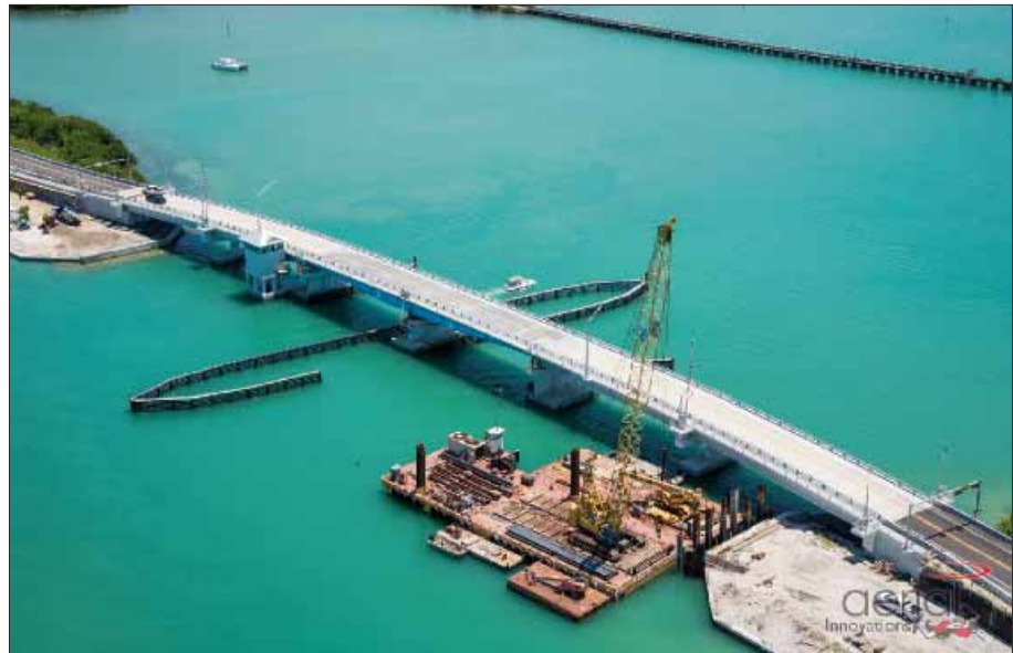
USA GRANDI LAVORI FINCOSIT Gasparilla Island Bridge Replacement
