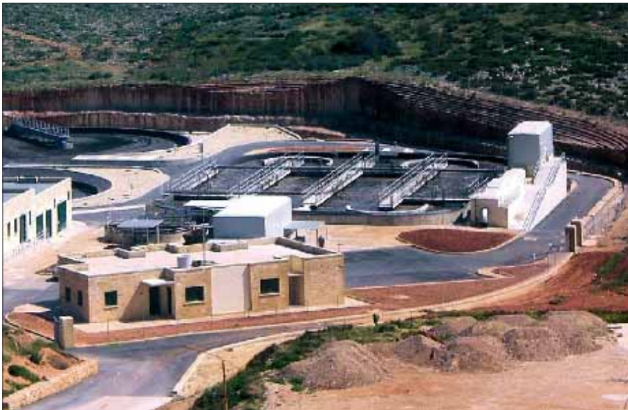
MALTA I.B.I. Waste Water Treatment Plant
