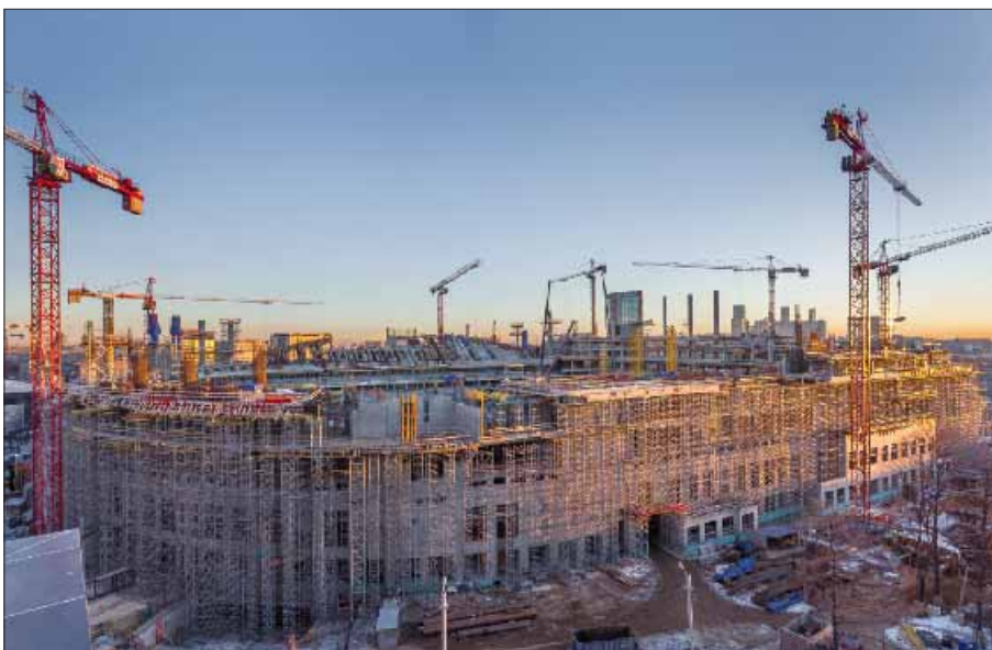
RUSSIA RIZZANI DE ECCHER VTB Arena park project
